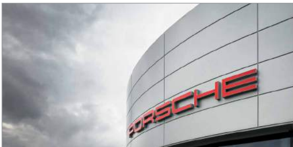
| Qbiss One, Metal Modular Façade System
